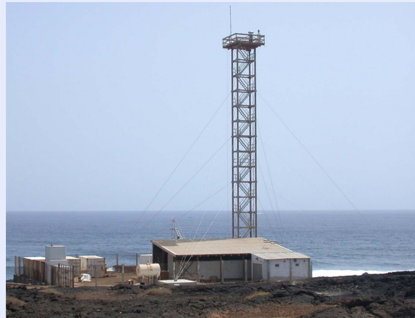
Fig. 1. Cape Verde Atmospheric Observatory (CVAO) with a 30 m-tower for aerosol particle sampling, ~100 m offshore.
